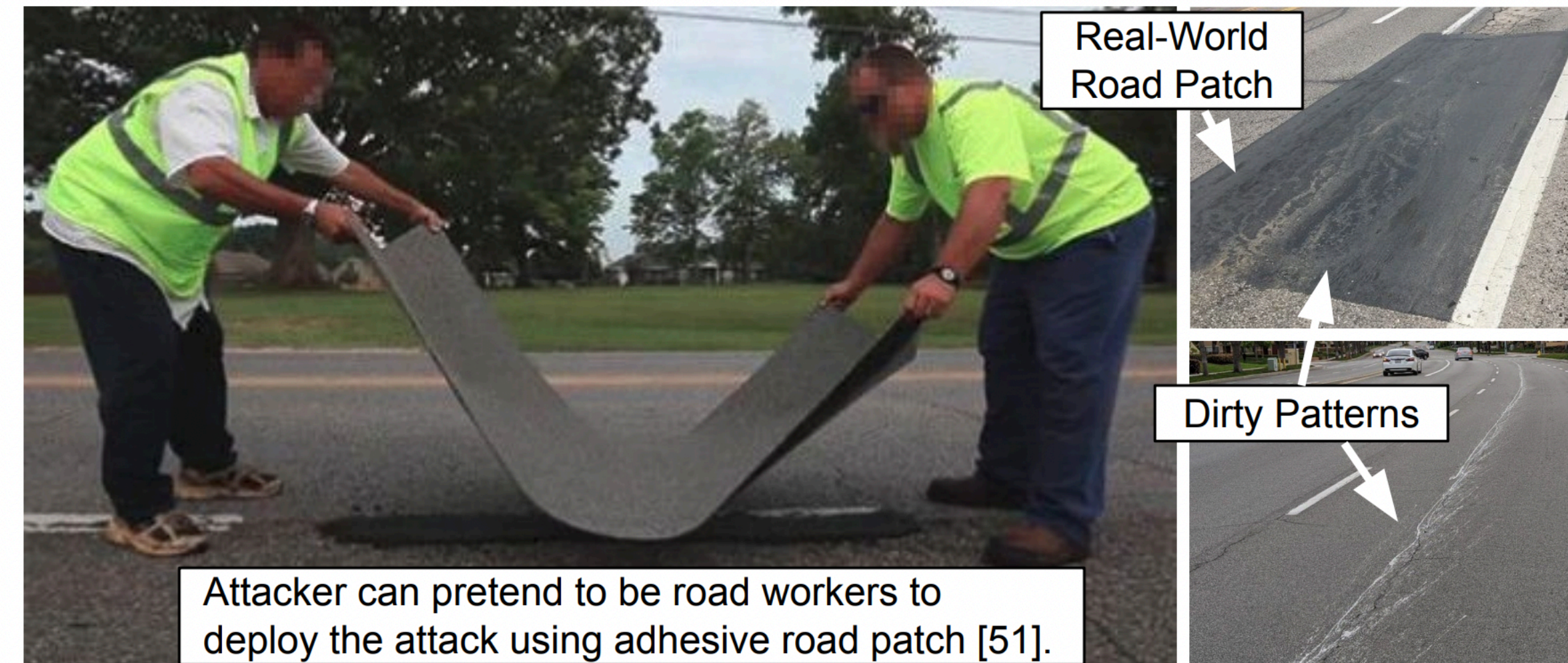
Figure 2: Illustration of our novel and domain-specific attack vector: Dirty Road Patch (DRP).
